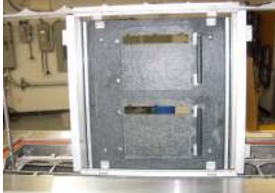
Photo 4 WSP after clean
